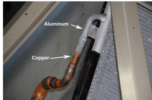
Figure 148: Connection Close-Up
