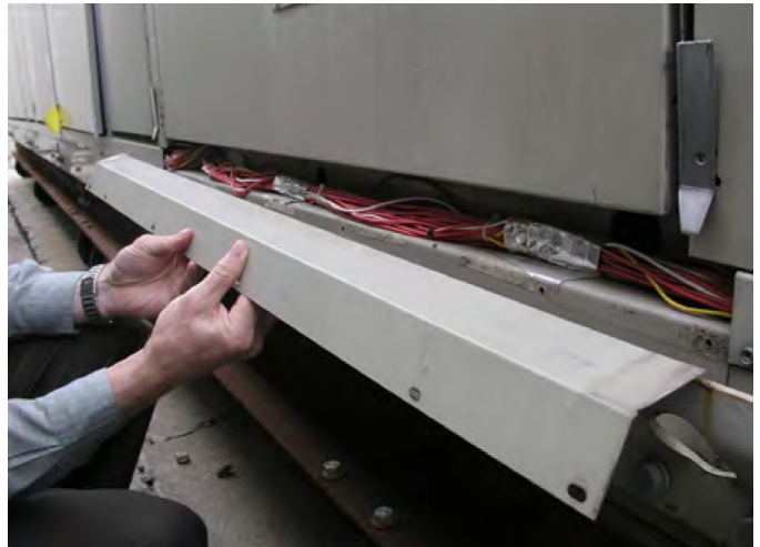
Figure 70: Control Wiring Raceway
