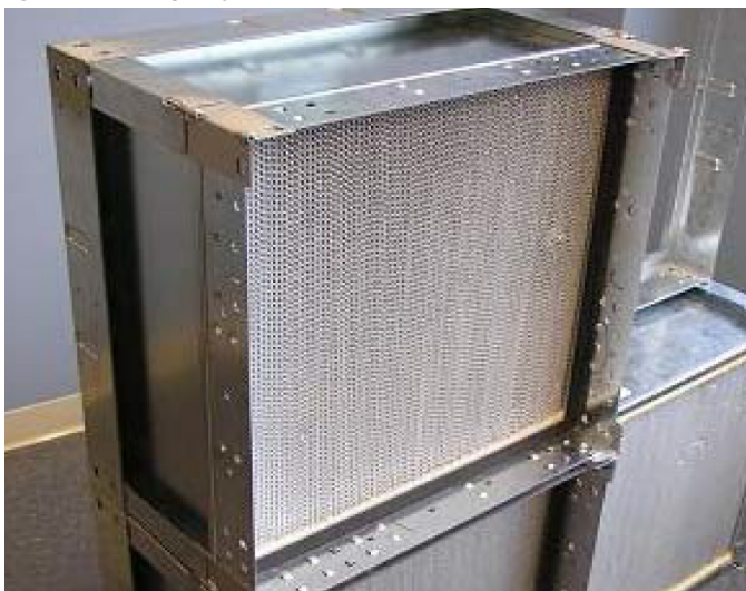
Figure 59: Properly Installed HEPA Filter
