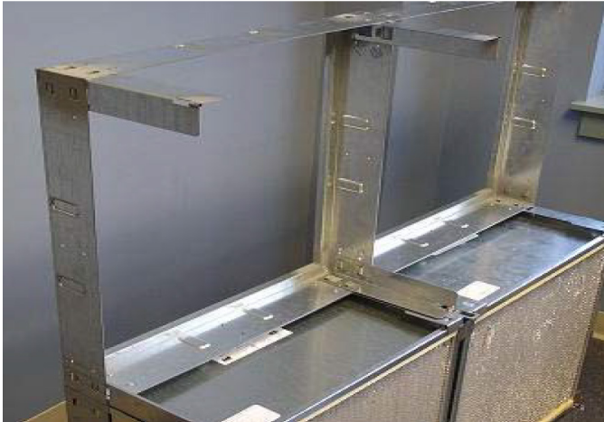
Figure 47: Frame with Leg Extensions Installed
