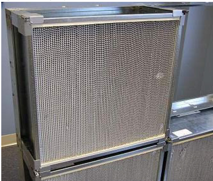
Figure 54: Properly Installed Filter Inside of the Frame
